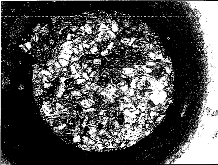
View of 7' diameter CDS separation chamber with a floating Styrofoam mat about 1' thick. Westlake System.
