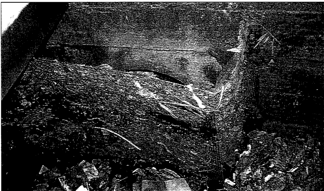
Vertical insert screen totally occluded with evidence of materials passing downstream. About 1"-2" of material on the floor of the catch basin.
