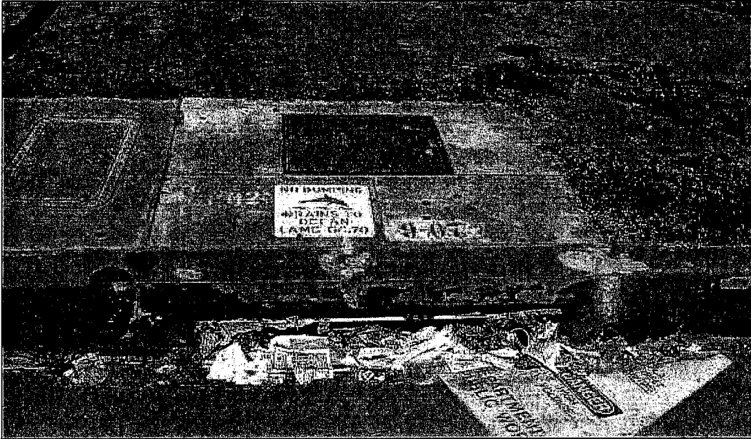
This retractable excluder is held open by trash which is jammed in the inlet opening.
