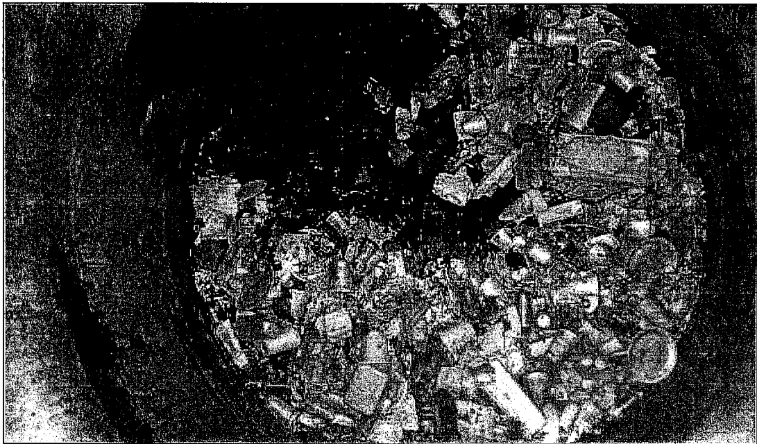
View of the separation chamber of the CDS system downstream of the catch basin retrofit study area. The mat of floating material is impenetrable past about 4' with a stadia rod. The unit appears to be full with approximately 10-14 cubic yards of trash, debris and sediment.
